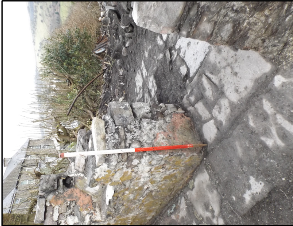
Plate 9. Oblique shot of northern reveal of rear doorway (view northeast)
