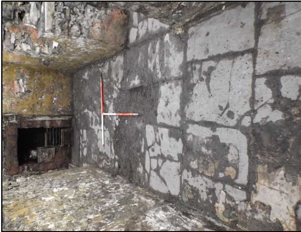
Plate 23. Remains of flagstone flooring with some remnant linoleum and bitumen to west of rear doorway (view north)
