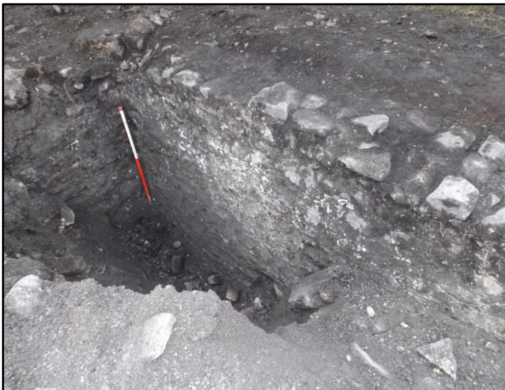
Plate 24. Western (front) elevation after partial clearance of later infill between pair of later partition walls (view southwest)
