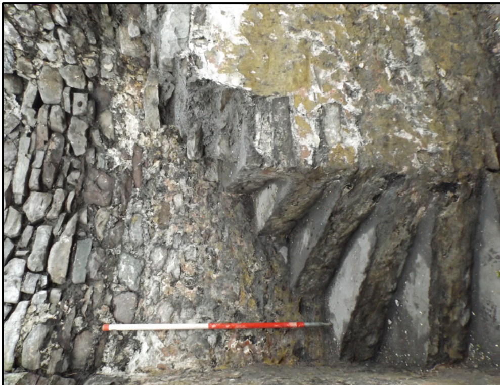
Plate 2. Staircase leading up west edge of fireplace, incorporated into north gable (view northeast)
