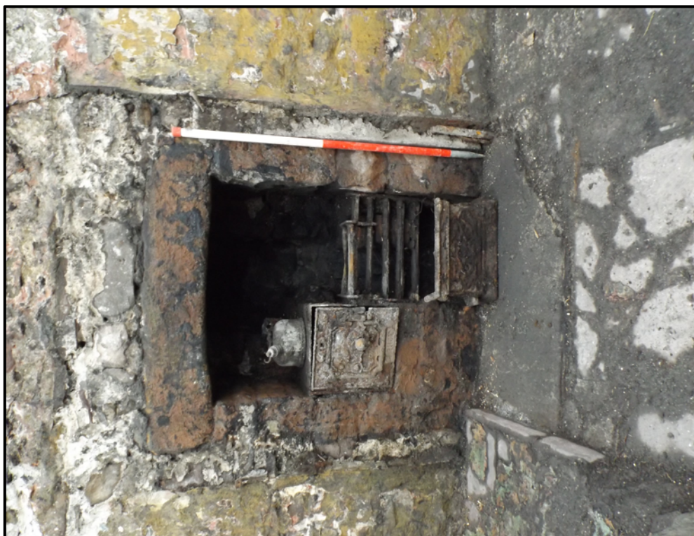
Plate 4. Fireplace incorporated into south facing north gable wall (view north)
