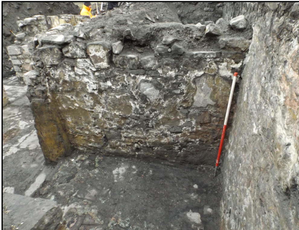
Plate 3. North-facing elevation of secondary partition wall abutting front (west) wall of house (view south)
