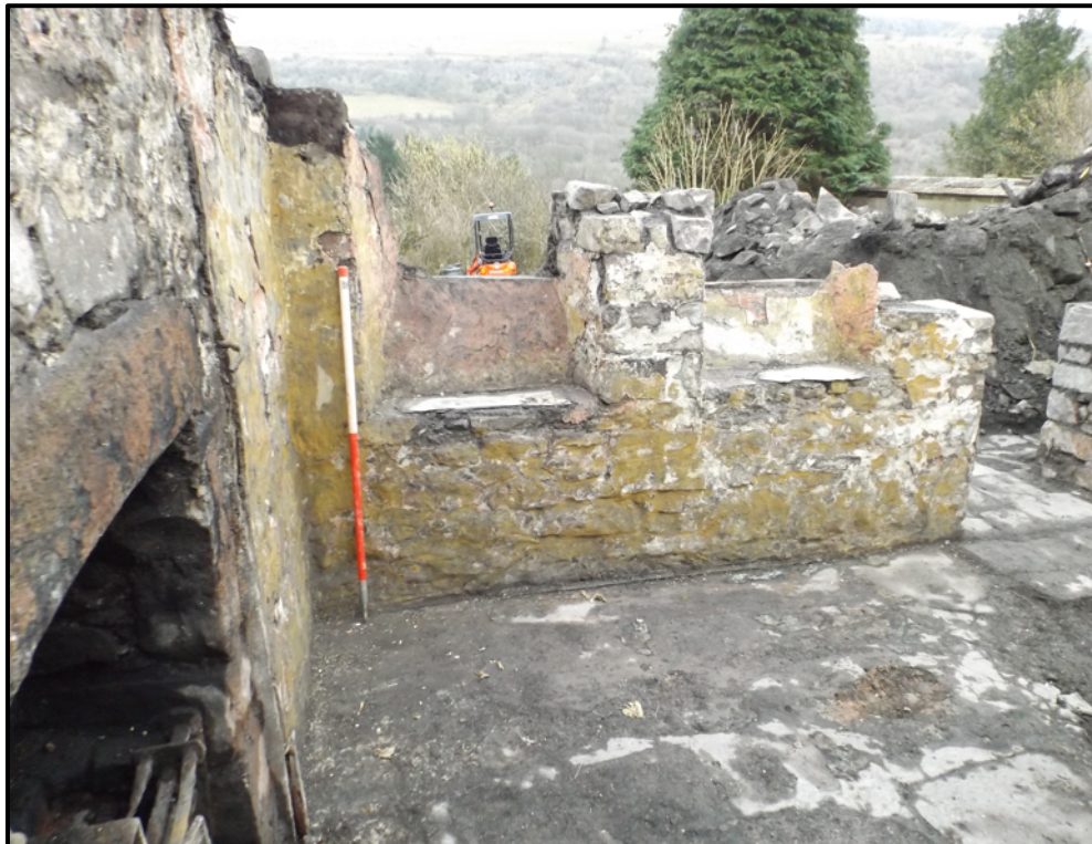
Plate 5. Interior view of light well windows in east elevation to north of rear entrance (view east)
