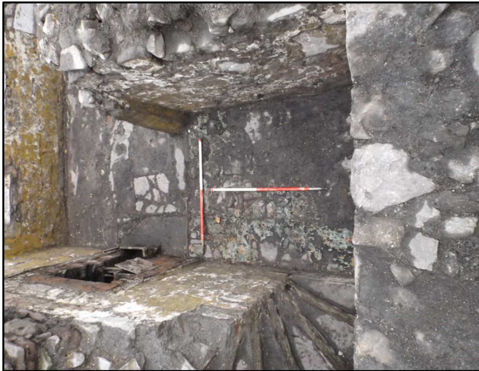
Plate 19. Remains of flagstone flooring and linoleum in area south of fireplace and staircase (view east)
