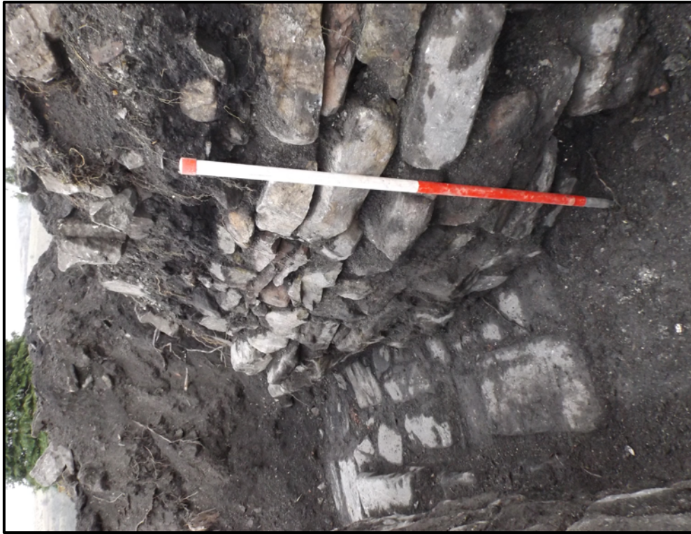
Plate 17. Oblique view of retaining wall to south of house's southern gable (view southeast)
