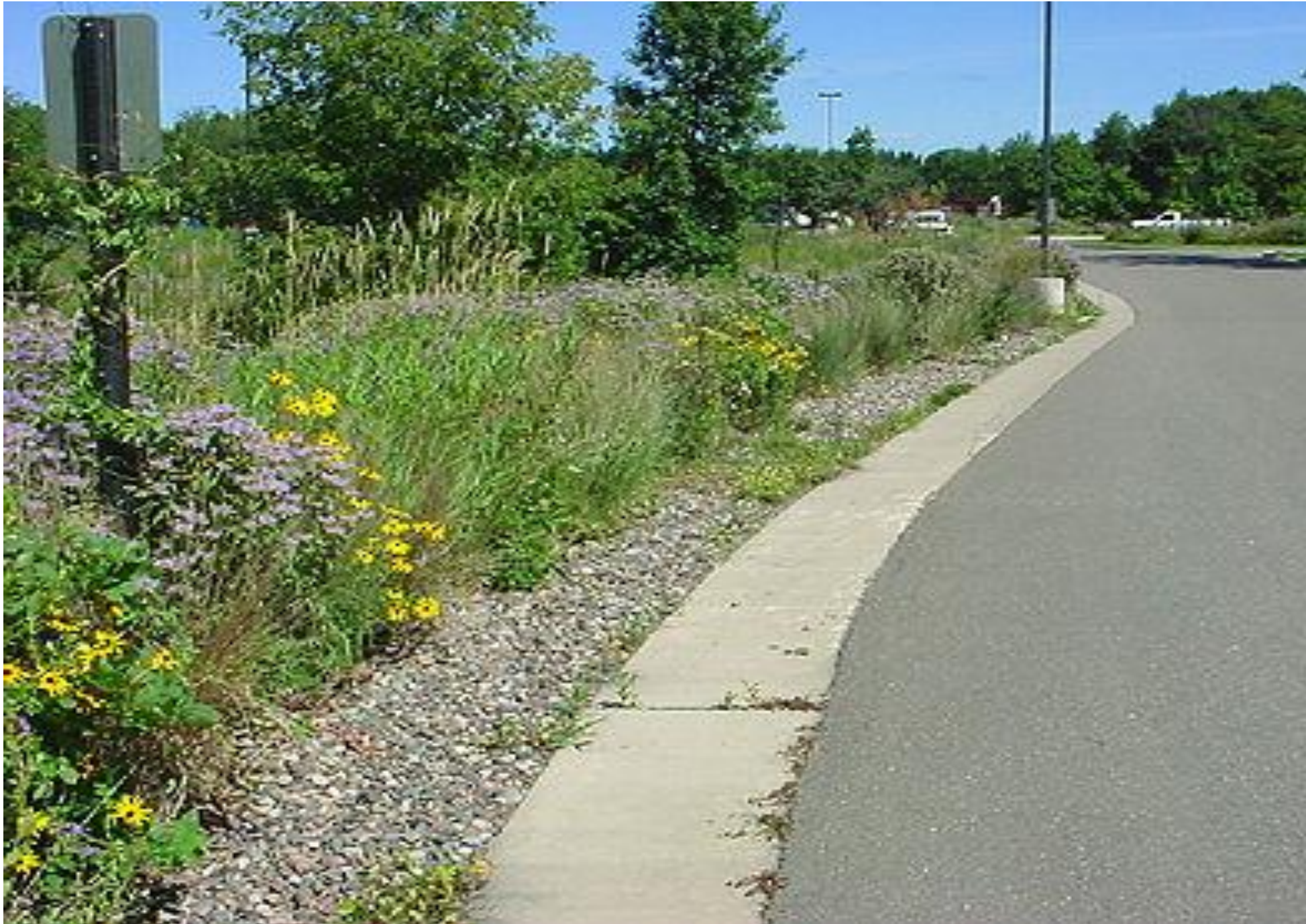
Stormwater Infiltration Trench
