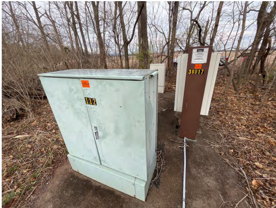
Photograph 44. View of buried, subsurface Verizon cables along Mountville Road.
