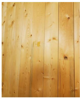
A CLT wall with finger joints
