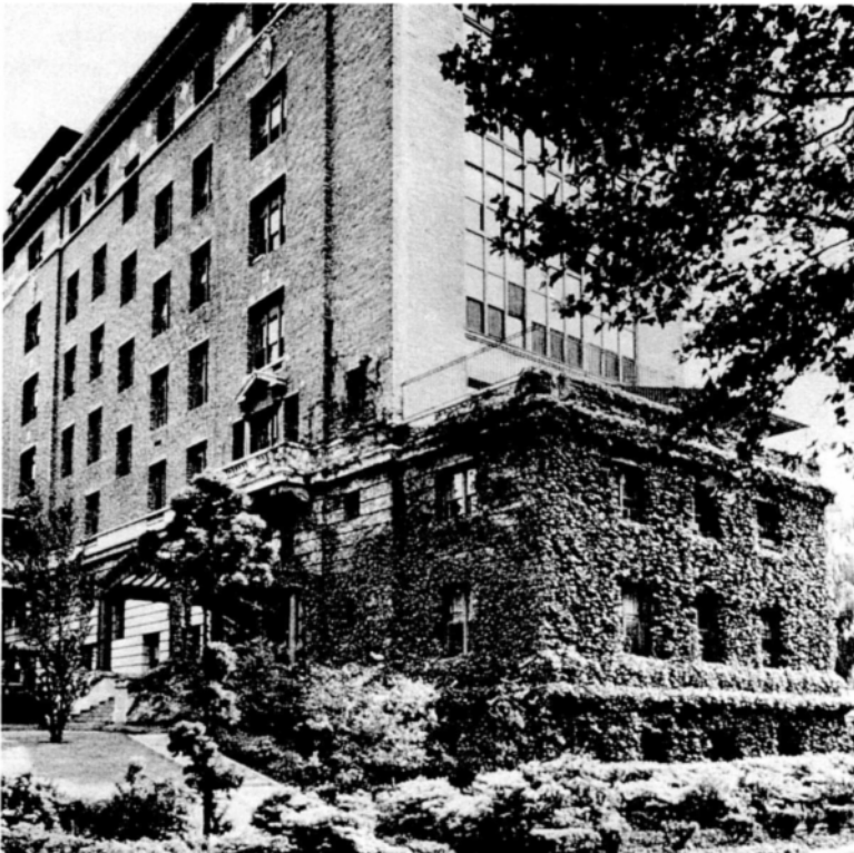
12 • The Hospital mellowed over the years as ivy began to cover its stark, utilitarian lines.
