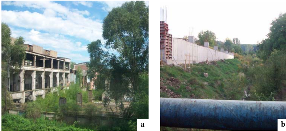
Fig. 3. Ruderale landscape – abandoned industrial property (a), interstitial spaces (b) Cluj-Napoca
