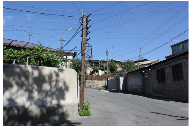
In Armenia, too, electrical poles are important connection points. Photo: P. Wind, 10-6-2014.
