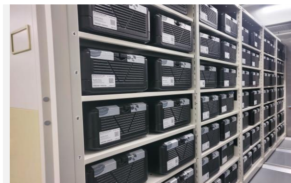
Figure - 3. The Storage room of BGSV
