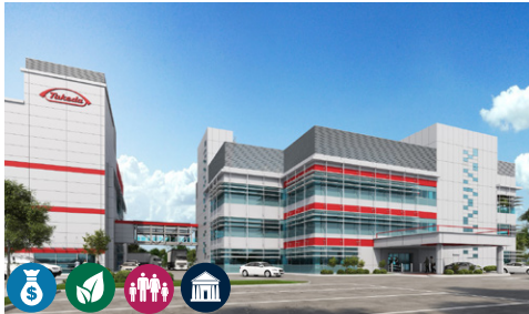
Takeda Singapore Biologics Manufacturing Support Facility
