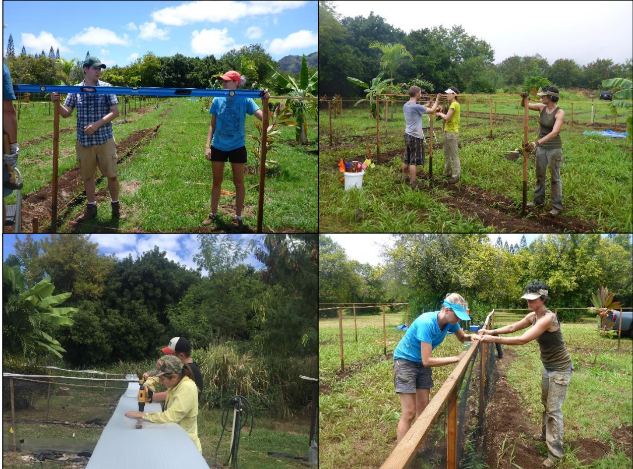
Figure 5. Clockwise from top left, with people identified left to right. Bob Thomson and Robyn Screen checking whether the heights of the upright posts are level. Anthony Barley, Rachel Goodman, and Laci Gerhart-Barley attaching the top frame (the bottom of third of the posts are darkened by copper paint). Robyn Screen and Laci Gerhart-Barley stapling mesh to the frame. You can see the berm of dirt that will be used to refill the trench. Stevie Kennedy-Gold and Marlin Dart attaching the top plastic (Solexx, note how it is one continuous sheet).
