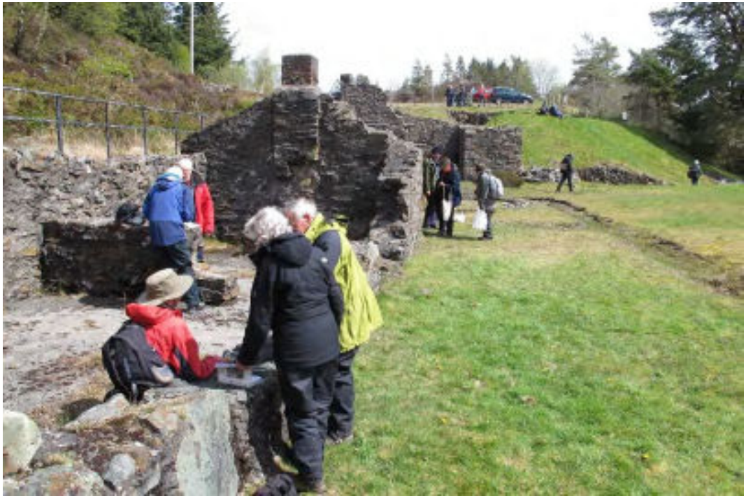
Studying the disused mine buildings at at Mwynylaudd. Image © Steve Price
