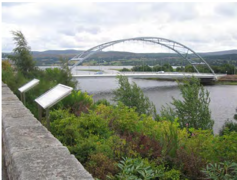
Bonar Bridge from the vc. 107 side, looking across into vc. 106. Phil Williams.
