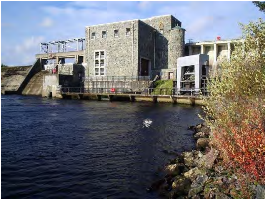
Lairg Power Station lies at the southern end of an extensive chain of major lochs. Donald Bain.
