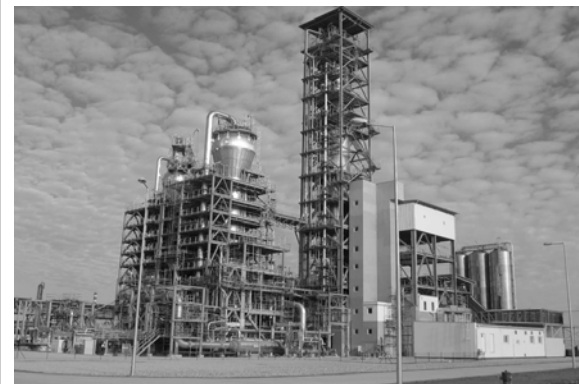
Slovnaft PP-3 plant
