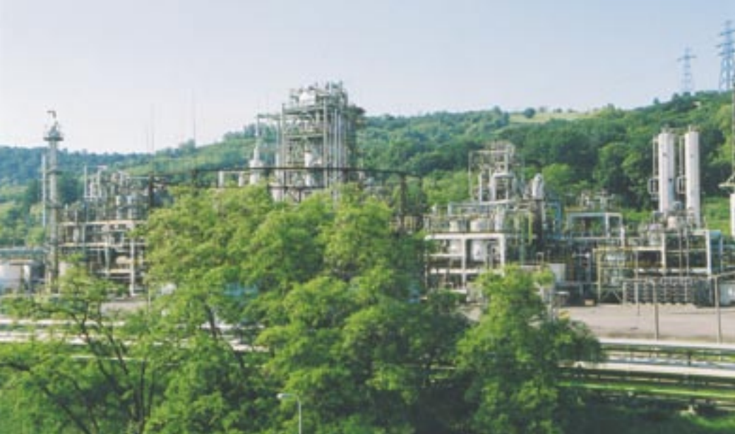
View of the MDI Plant
