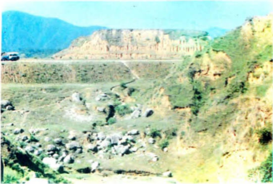
Degradation of vegetation and land as a result of developmental activities (construction of dam and canal for Pandoh hydroelectric project, Sundarnagar, Kullu)
