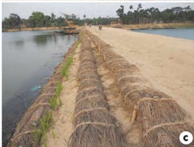
a. Sand erosion of boro bandh on Mundeshwari river at Chingra, Khanakul, Hooghly; b. Habit of Saccharum bengalense (inset: Bundles of culms); c. & d. Hete arranged and fixed to prevent sand erosion
