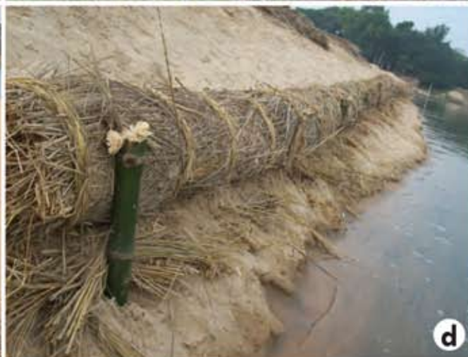
a. Sand erosion of boro bandh on Mundeshwari river at Chingra, Khanakul, Hooghly; b. Habit of Saccharum bengalense (inset: Bundles of culms); c. & d. Hete arranged and fixed to prevent sand erosion
