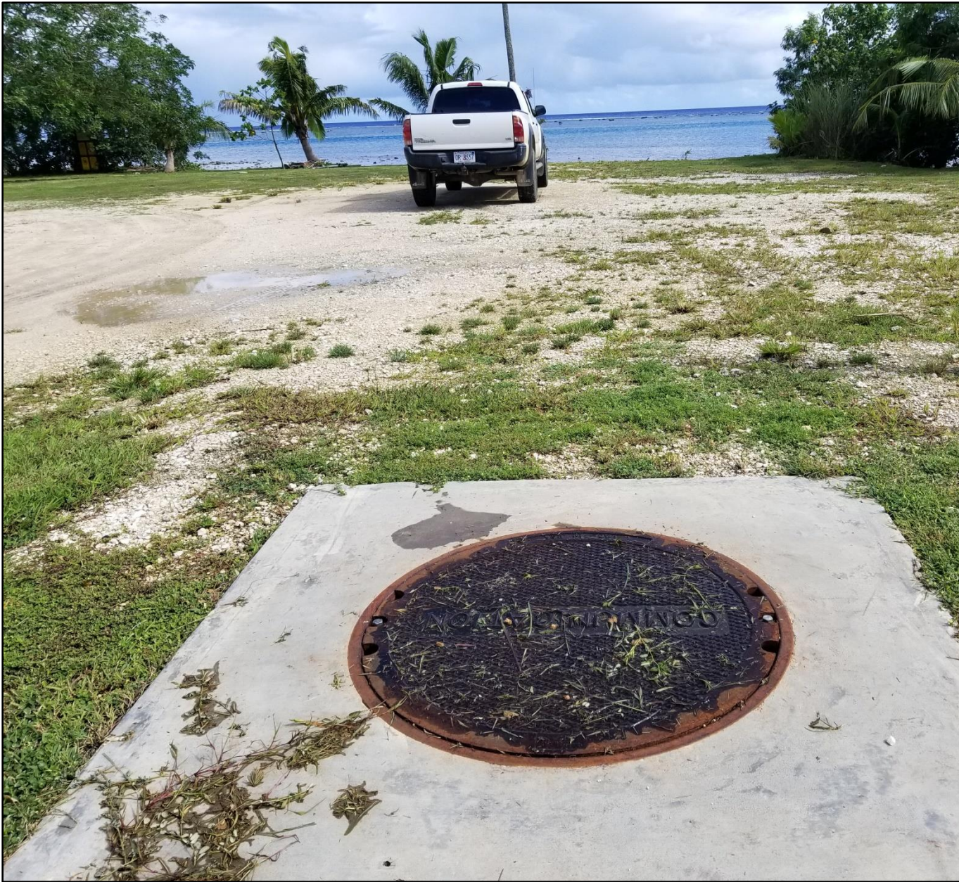
Photo 2. GTA Beach Manhole installed in 2017 located within Santos Park, facing north.
