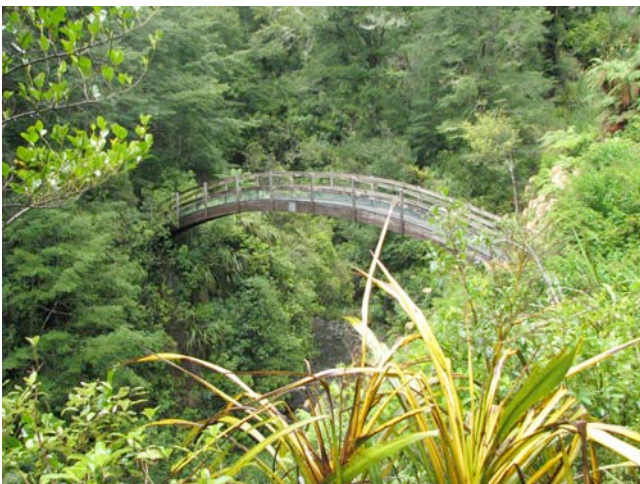
Fig. 8. Umutoi River bridge, Ruahines, 18 Jan 2009. Photo: M.D. Wilcox.
