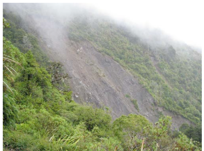
Fig. 10. Rangiwahia Track, slip, 19 Jan 2009. Photo: M.D. Wilcox.
