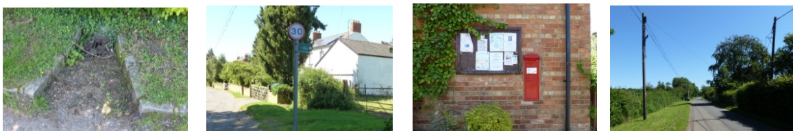
Stone lined gutters, highways signage, street furniture and telegraph poles in Singleborough
