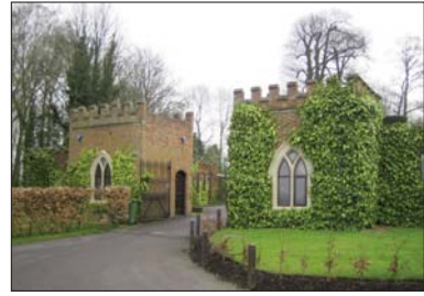
Parapet roof
