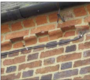
Dentilated brickwork
