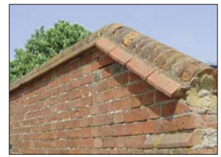
Spalling brickwork
