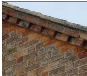
Dentilated brickwork
