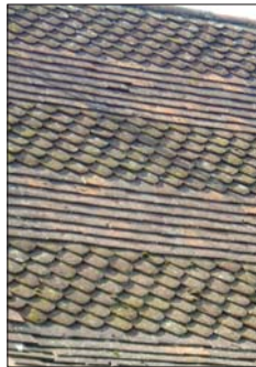
Decorative tiled roof
