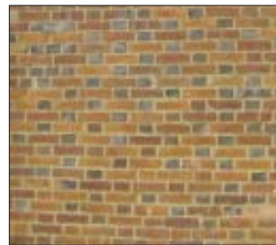
Flemish Bond with vitrified headers
