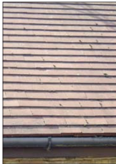
Modern machine made tiled roof
