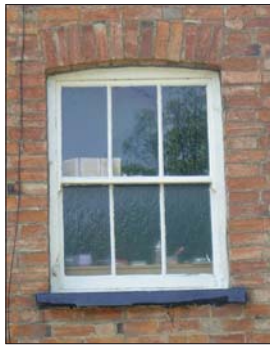
Bricked arched lintel
