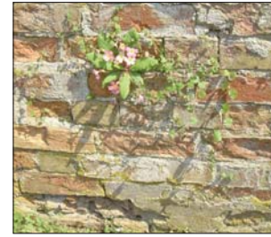
Spalling brickwork
