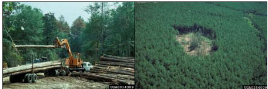
Figure 11. Tree felling is a control method (left) used to prevent expansion of spot infestations (right, spot after infested trees have been removed). Infested trees and uninfested trees in a buffer zone are either cut and removed or cut and left in place, in either case for the purpose of stopping spot expansion. (Both photos: Ronald F. Billings, Texas Forest Service, Bugwood.org)
