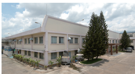
■ PLUS VIETNAM Plant No.1 (Bien Hoa Plant): Approximately 26,400 m 2
