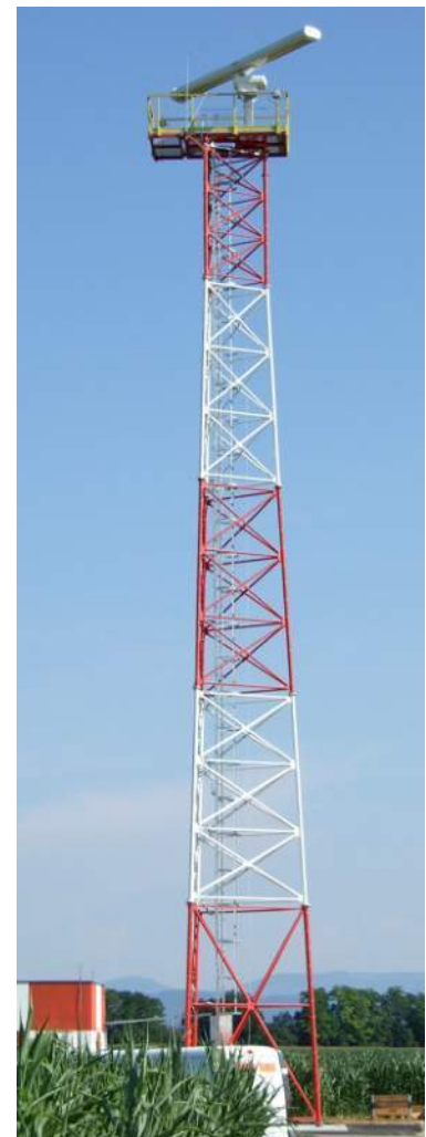
Figure 7.1 Three-legged lattice tower
