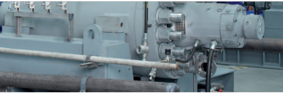
KSB employees install the piping of a boiler feed pump.
