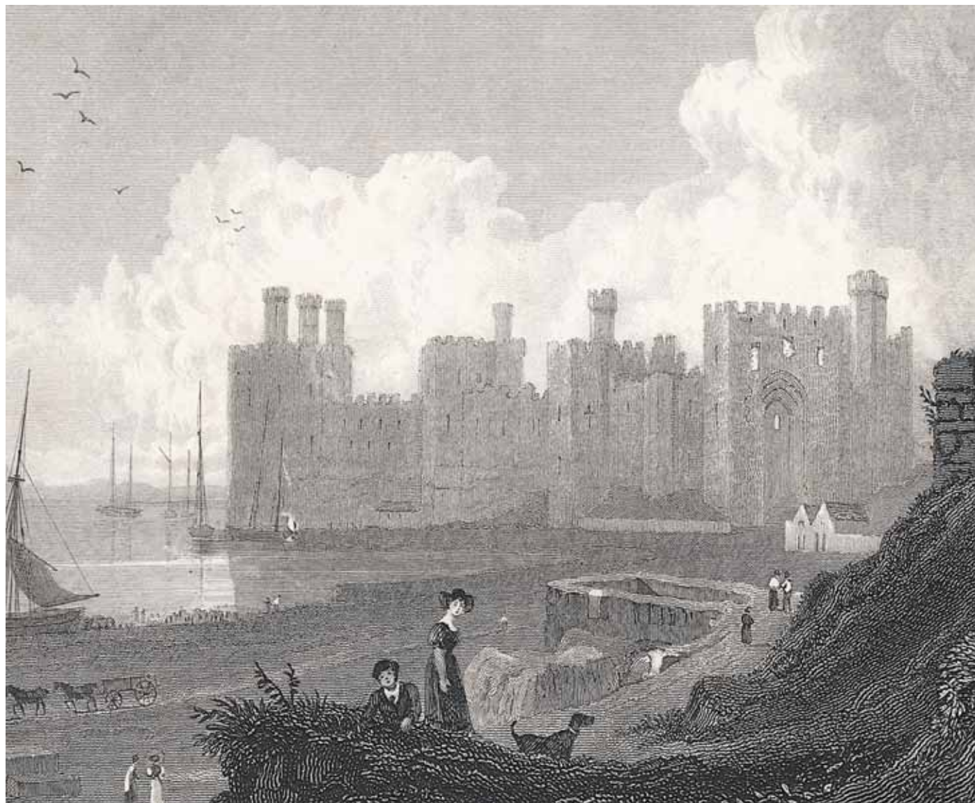
The Slate Quay consolidated the informal shore of the Seiont in the early nineteenth century (Henry Gastineau, Caernarvon Castle, about 1830–40, The National Library of Wales).
