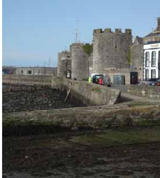
Jetty and slipway at the limit of the medieval quay.
