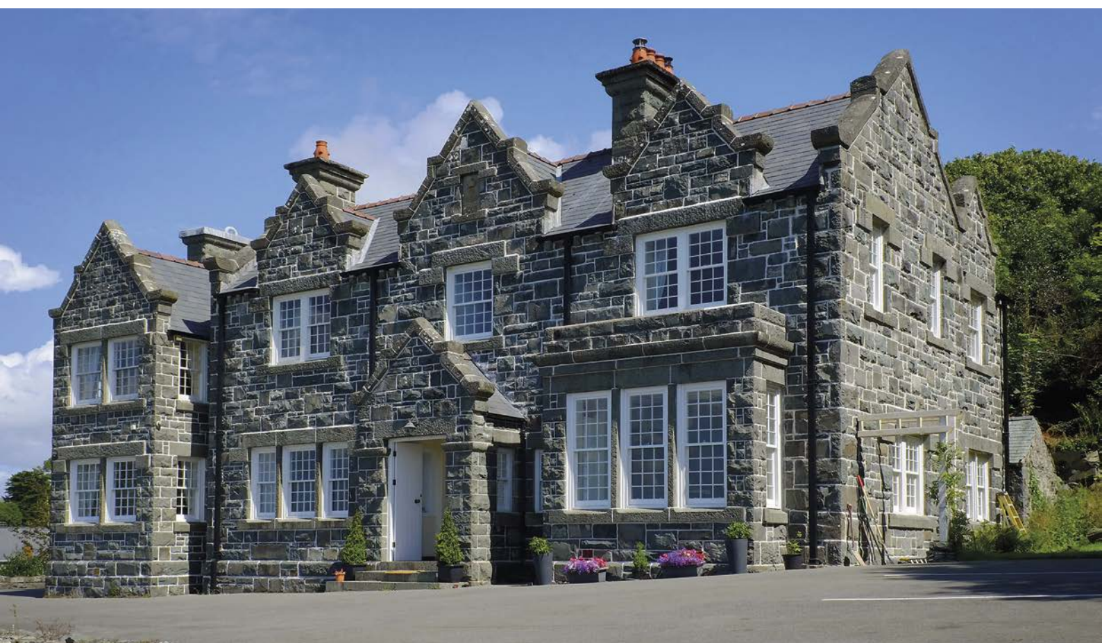
Crown Lodge, also designed by George Walton, has a rugged finish favoured by Arts and Crafts architects (© Copyright: Crown Lodge, Harlech).
