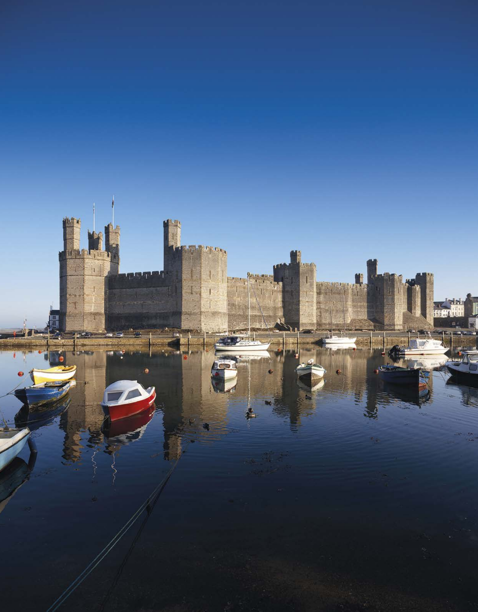
Monitoring the implementation of the management plan includes the Cadw annual and quinquennial inspections of the six ancient monuments. Various repair works to Caernarfon Castle were identified as necessary in the 2016 inspection.
