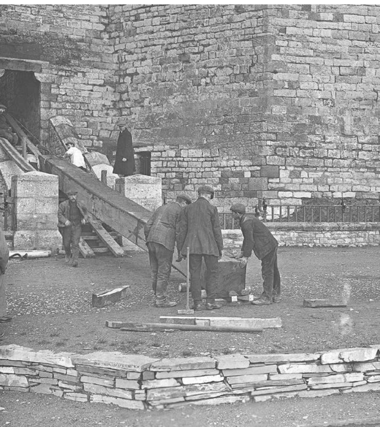
Restoration work at Caernarfon at the beginning of the twentieth century. Here, a massive oak beam is being brought into the castle from the quay echoing centuries of building practice.
