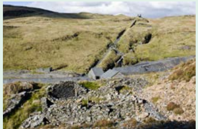
Above right: Winding house, Rhiwbach Quarry, Gwynedd. © Crown copyright: RCAHMW
