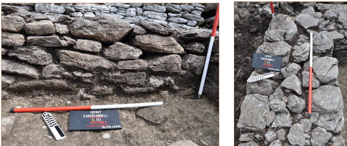
Fig. 30 Coursed section of house wall.
