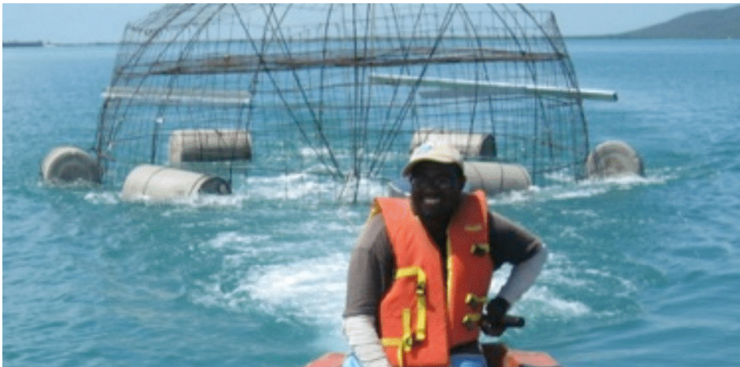
Towing an artificial reef into position
