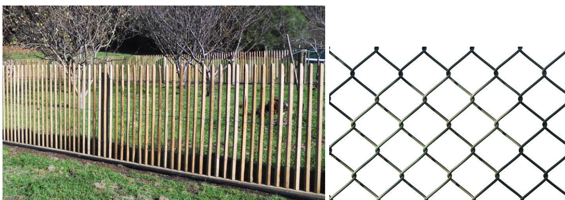
Figure 17. Suggested fencing showing wood latte for aesthetic appeal, approximate spacing so the wetland is visible, and diamond mesh which must be on the inside of wooden latte.
