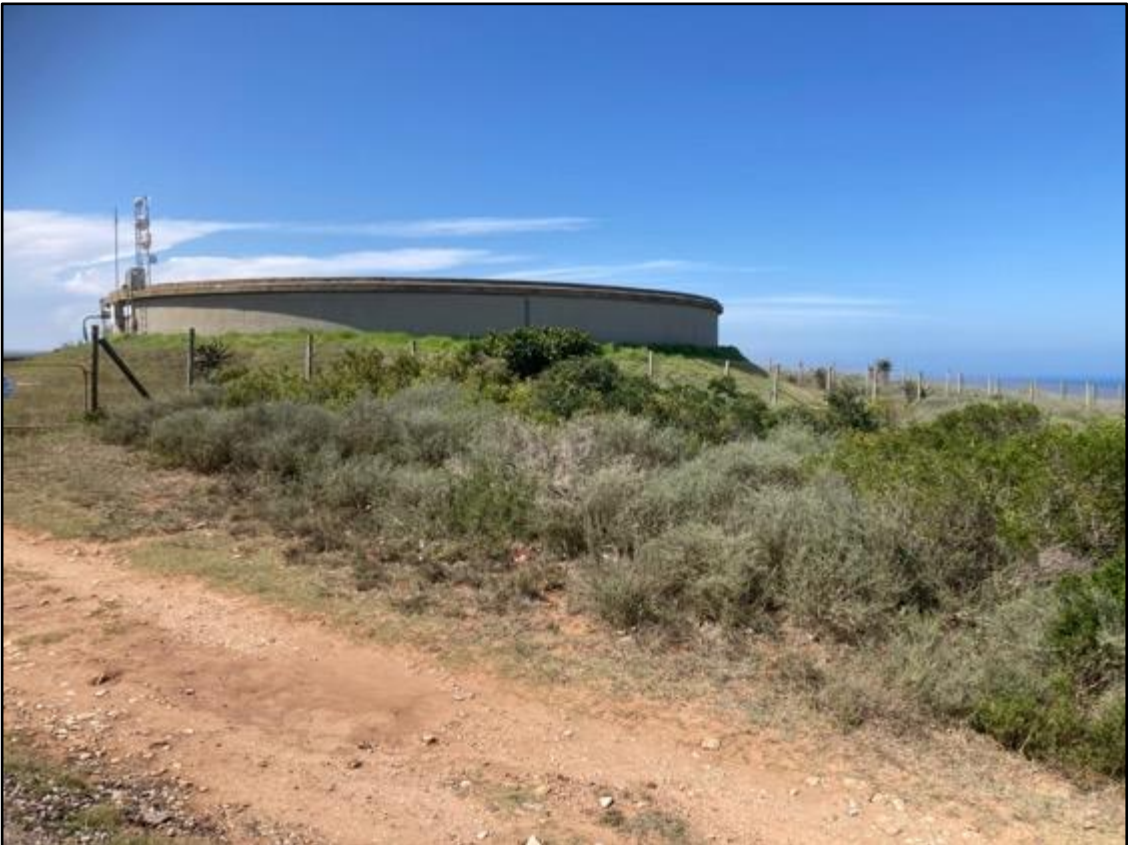
Figure 15: Reservoir in centre of property.
