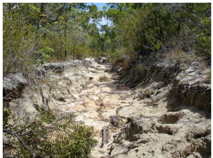
Figure 3.82 Firebreak erosion – A Mount Cook Firebreak eroded 1.5 metres after 1 wet season
