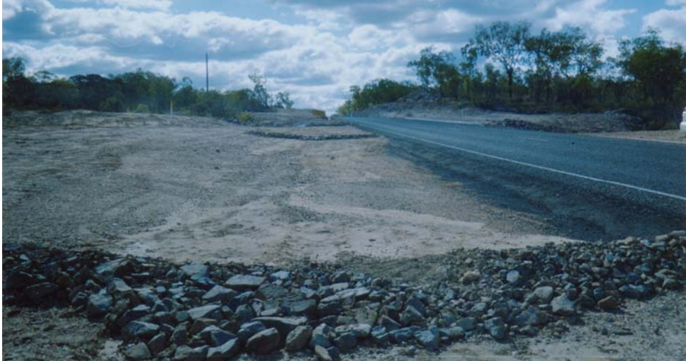
Drainage control improvements on the Lakeland - Laura Road
