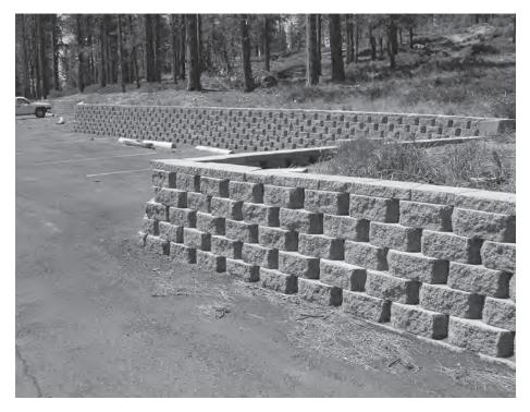
Photograph HD/22. New stone parapet wall along parking lot in front of concessionaire dorms.
