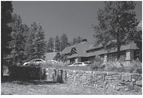
Photograph A/9. The retaining wall between the Lodge and the Sunrise Motel Unit which creates the space for the Registration Parking Area.
