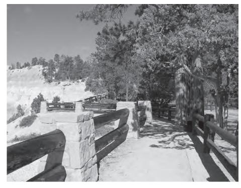
Photograph RT/16. "Primary Barrier" - wooden log fence with stone piers and "Secondary Barrier" wood log fence along Rim Trail.
