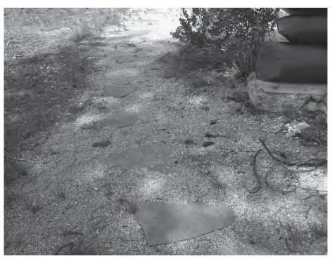
Photograph GS/14. Path around Old Administration Building with irregularly-shaped stone treads set in gravel.
