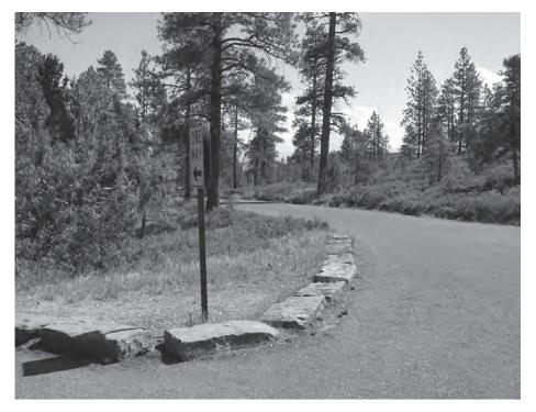
Photograph GS/13. Rugged stone curbing along road edge.
