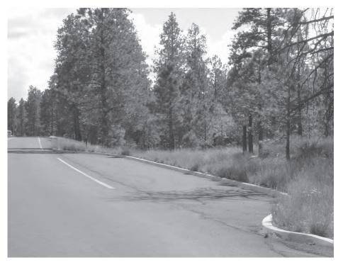
Photograph RR/8. Concrete curbing along pull off on Rim Road.
