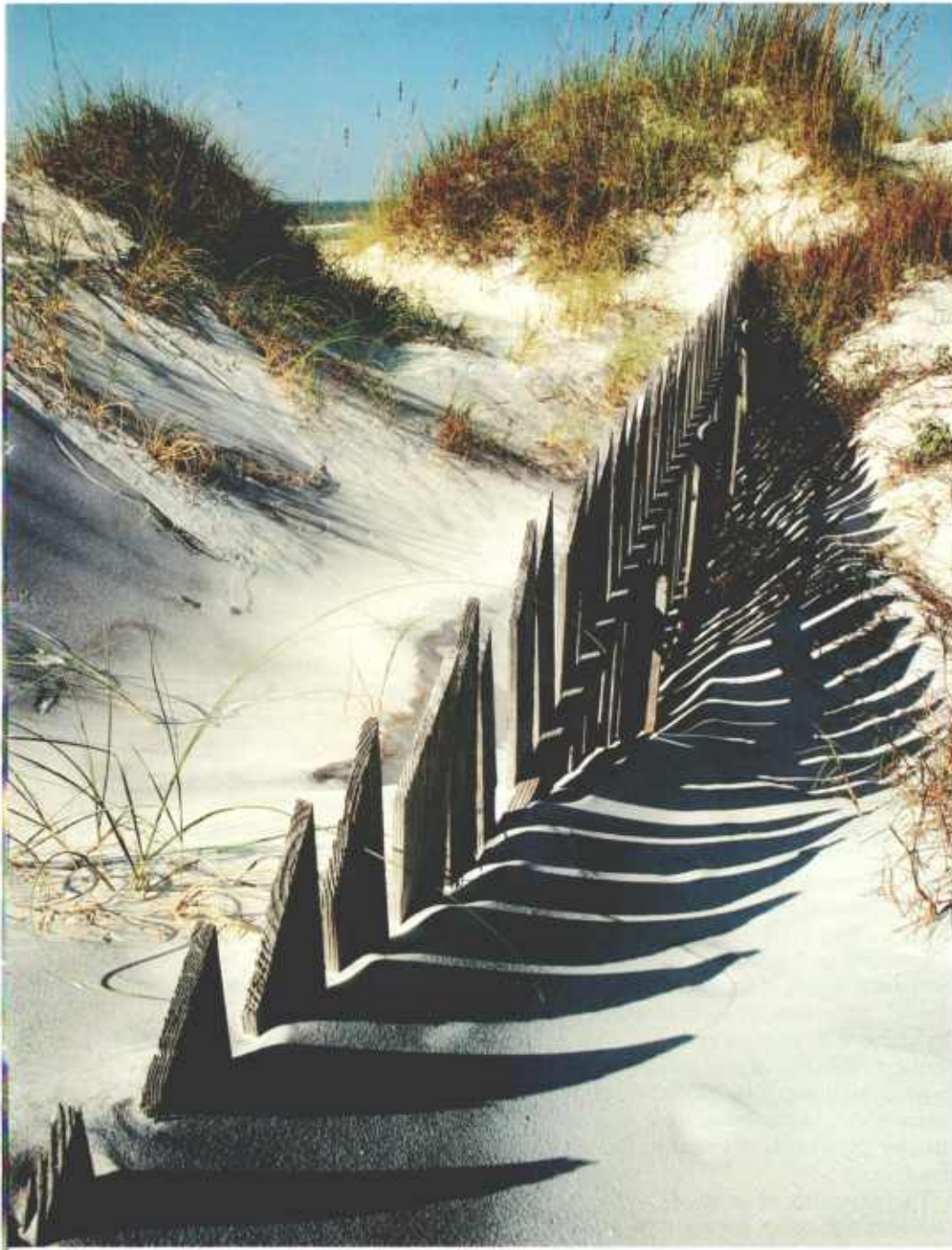
The near-burial of this sand fence is proof of its effectiveness in building dunes.
