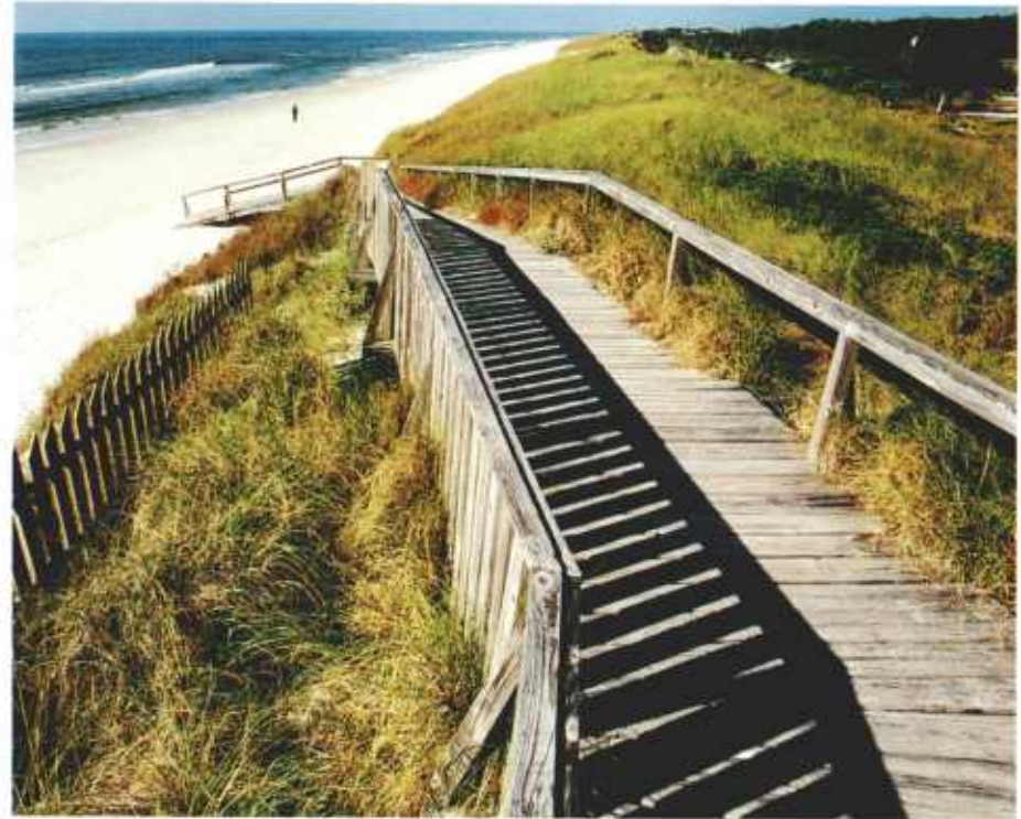
An example of well-planned dune protection: a dense cover of adapted grasses and a walkway that allows access to the beach without endangering the dunes.
