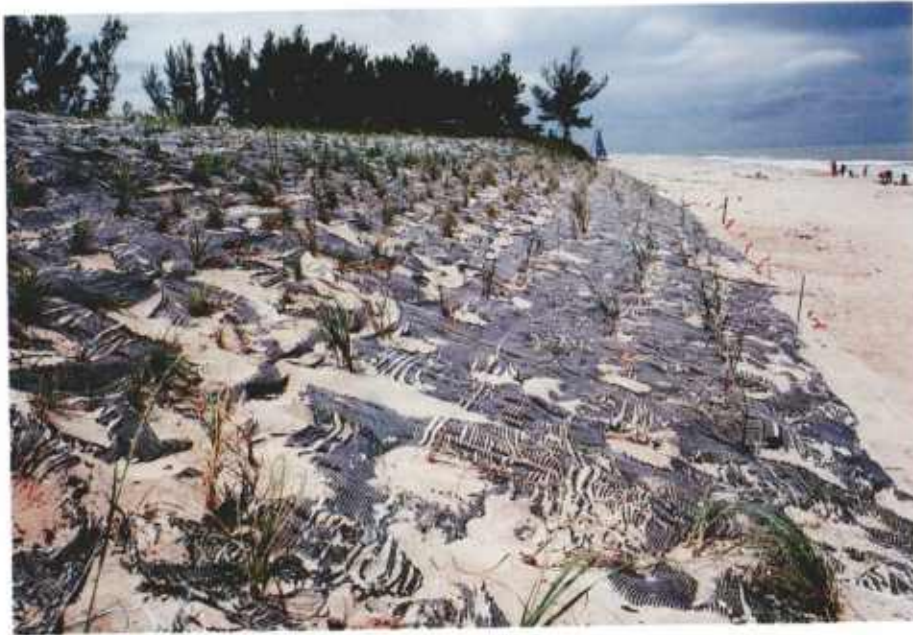
This new planting of sea oats and seashore paspalum is protected by an erosion-control fabric made of plastic netting interwoven with strips of paper.
