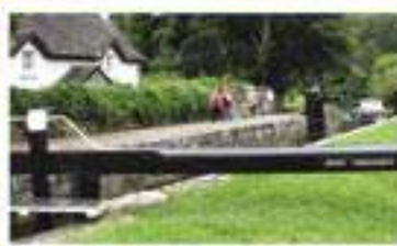
The Barrow Way at Tinnahinch Lock
