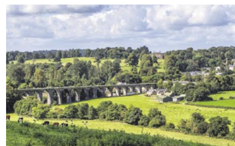
Borris town and 16-arch viaduct
