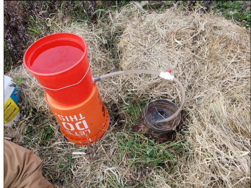
Photo 28: A double ring infiltrometer used to confirm that substrate on Work Pad #3 is much less pervious than natural hilltop soil. 11-11-19.
