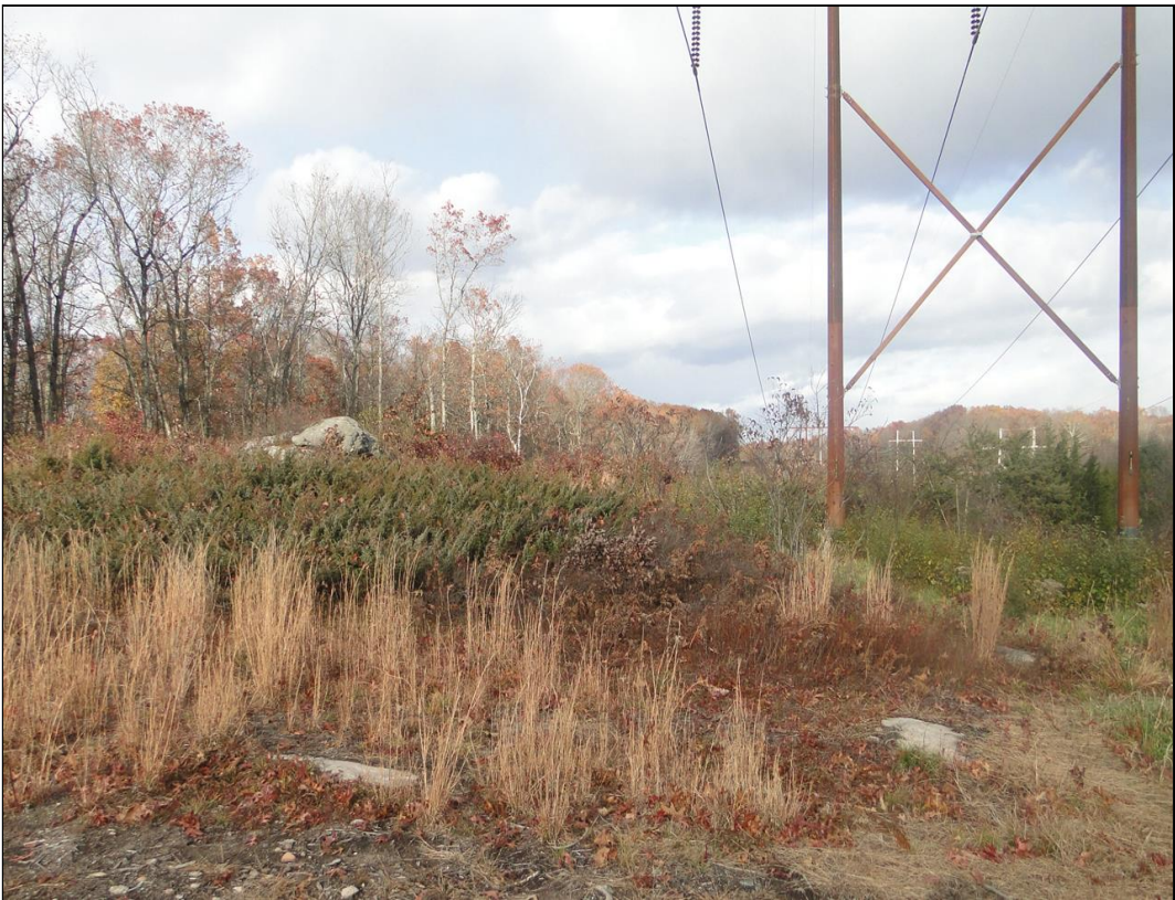
Photo 31: Northwesterly view of Pad #4. Heavy equipment clearly operated from this side. Permeability was good, averaging 0.56 minute for each 1" drop in water level.
