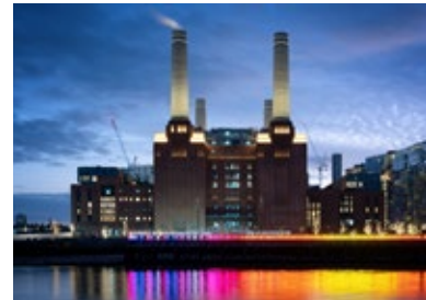
BATTERSEA POWER STATION SEEN FROM THE NORTH SIDE OF THE RIVER THAMES
