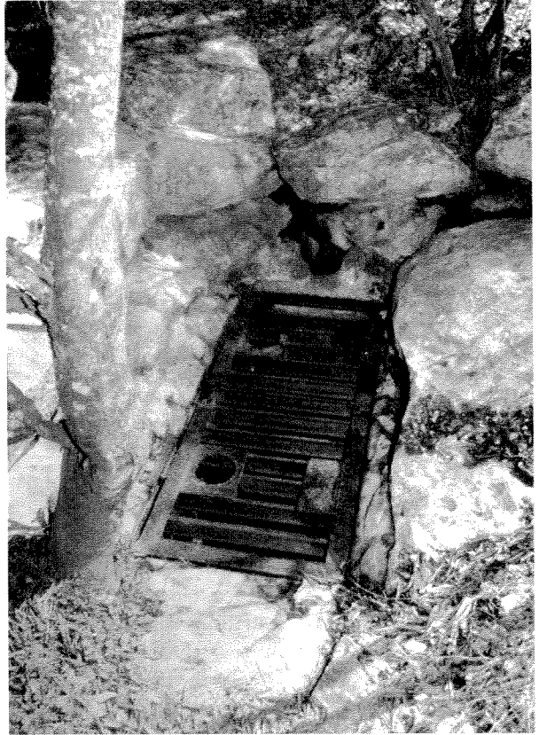
Fig. 34.5. A strong cave gate on the entrance of Lakeline Cave, Texas; length about 2 m. The gate has shielded hinges and two locks for greater security. Note the animal access hole through the ledge, which provides access to raccoons and mice. Photo by William R. Elliott.
