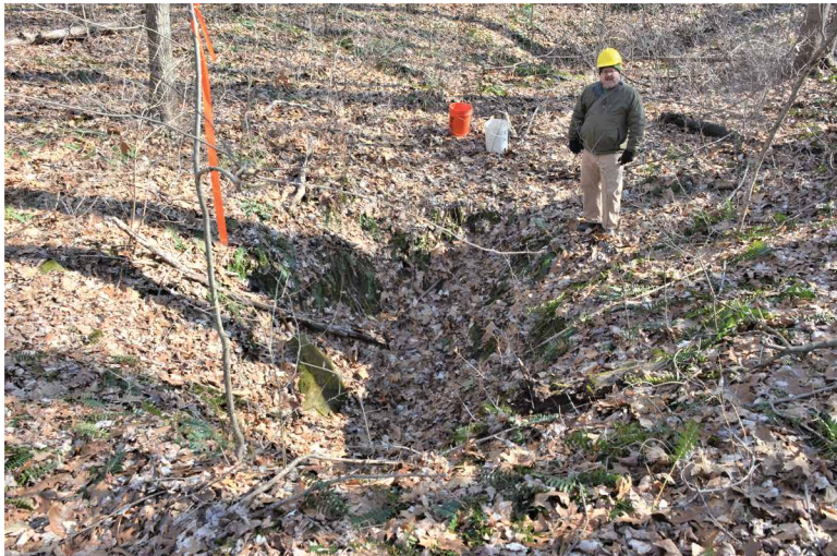
Figure 4. Kimball Tract sinkhole 1.
