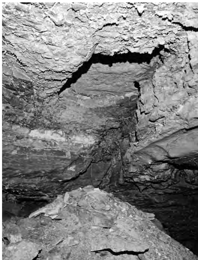
Figure 8. A ceiling breakout forming a rubble pile of rock fragments and rock flour.
