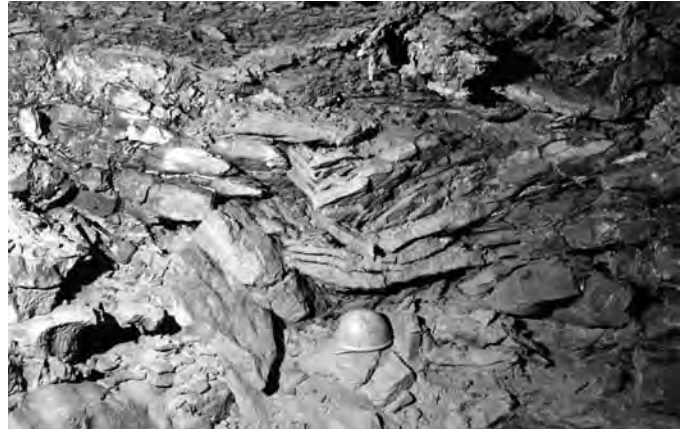
Figure 1. Rubble wall caused by gypsum deposition along bedding planes. Note hardhat for scale.
