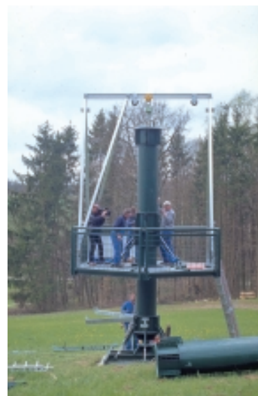
Fig. 74. Manual erection of the COPAS masts in Ulm.
