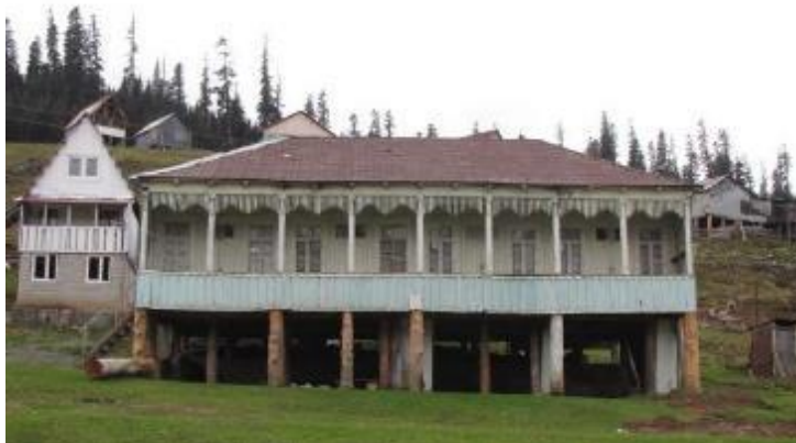
Former Pioneer Camp building in Bakhmaro
