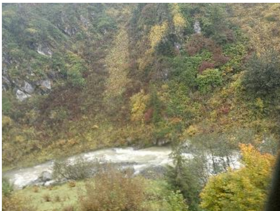
Figure 3.1.4.1. View of headworks location
