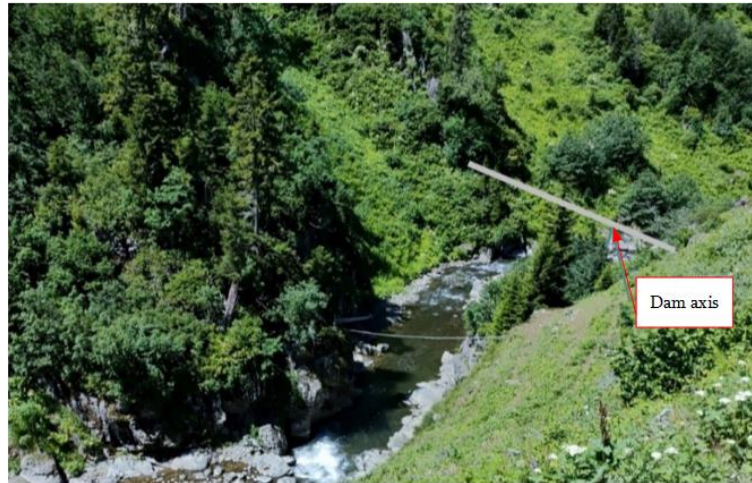
Figure 5.2.2.8.1. View towards proposed weir location
