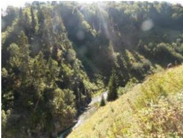
Headwork Alignment View
