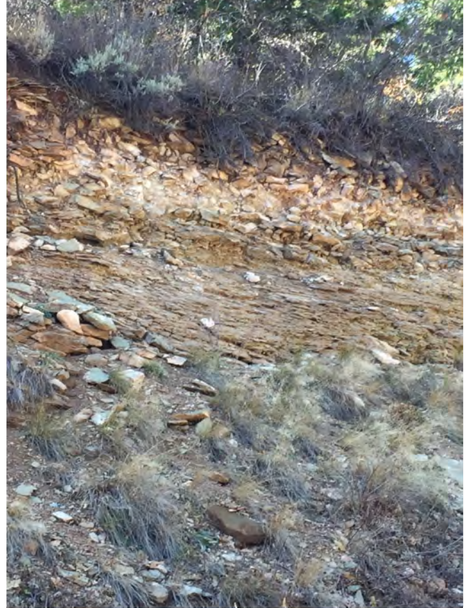
Highly fractured, horizontally bedded sandstone at Brusher Canyon service road off East Canyon Road
