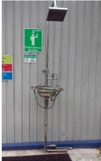
Figure 5.5 – An example of an emergency shower with an eye washing unit
