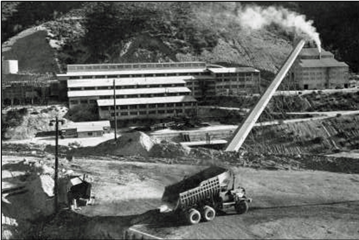
Figure 86. Castle Dome concentrator, circa early 1950s (photo from Arizona Geological Survey)
