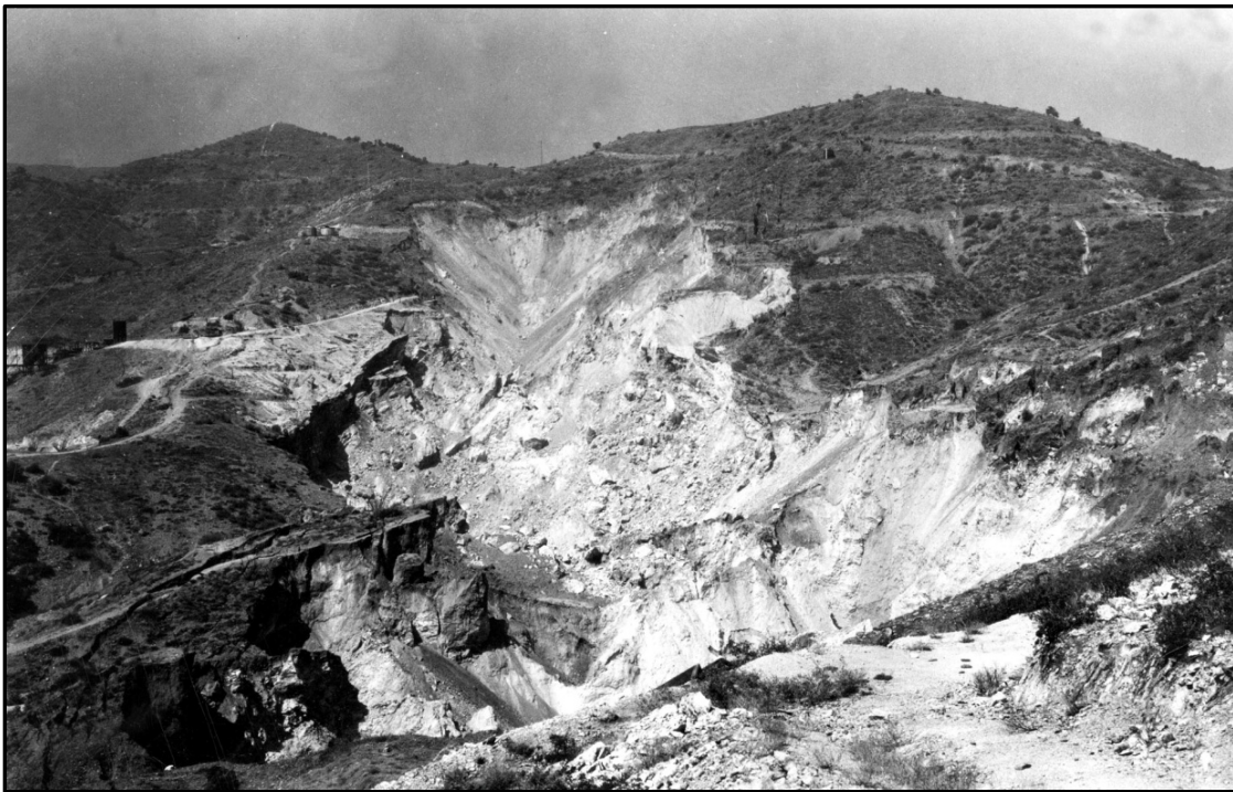
Figure 74. Subsidence above the Joe Bush ore zone, circa 1919 (photo from U. S. Geological Survey)
