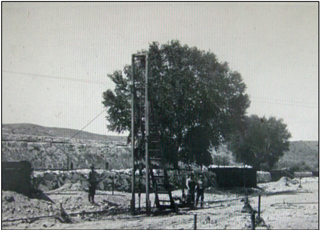
Figure 107. Churn drill along Pinal Creek near the Old Dominion mine, circa 1916 (photo from Gila County Historical Museum)
