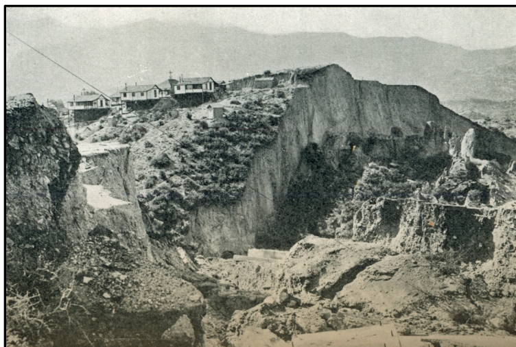
Figure 59. Dramatic effects of subsidence resulting from underground mining operations at Miami (photo from Parsons, 1933). When mining ceased in 1959, the zone of surface subsidence measured 3,400 feet north-south by 2,600 feet east-west and was more than 400 feet deep (Burgin, 1976)
