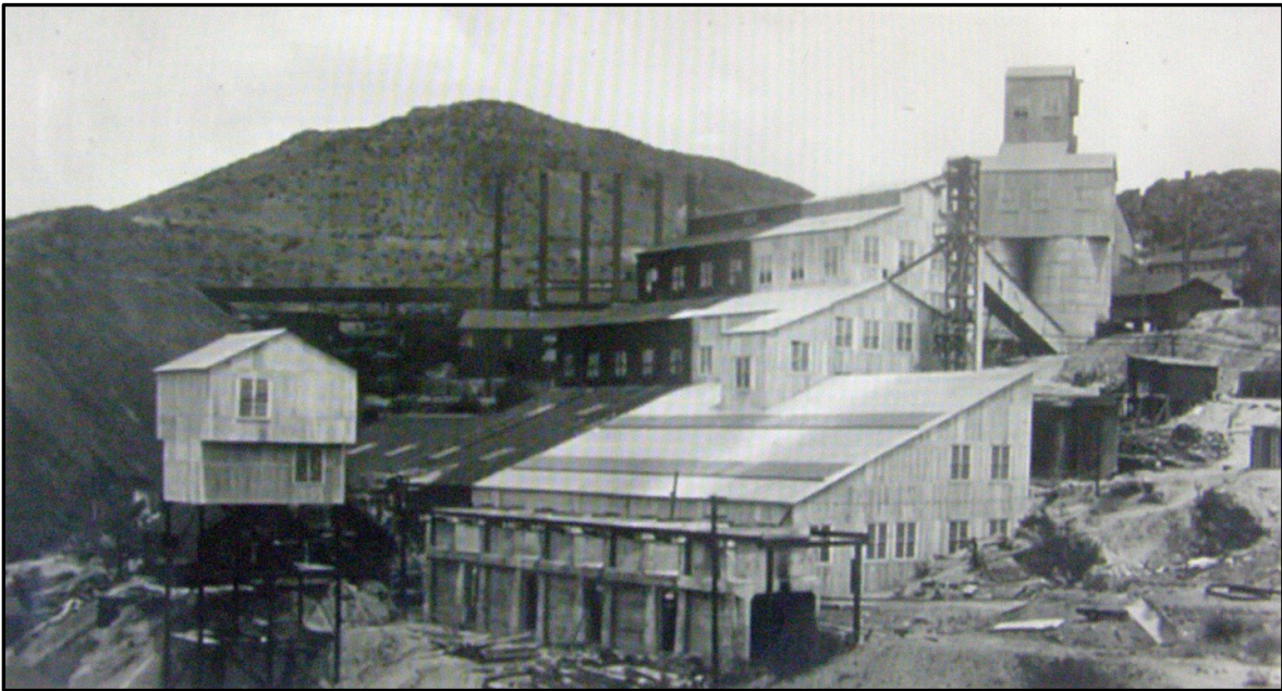
Figure 39. Old Dominion concentrator, circa April 1914. Note: Like many mills, both past and present, it was located on a slope of a hill, which allows gravity to move the ore from one stage of processing to the next (photo from Gila County Historical Museum).
