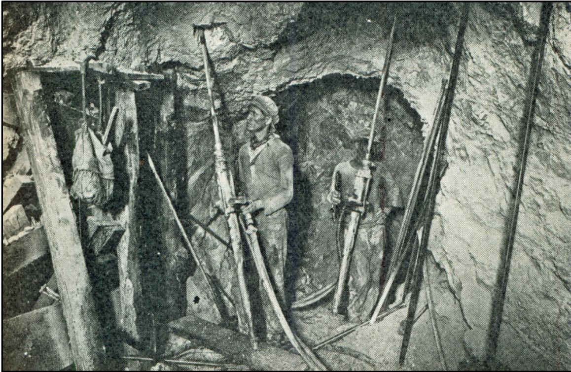
Figure 60. One-man pneumatic drills at Miami (photo by Parsons, 1933)
