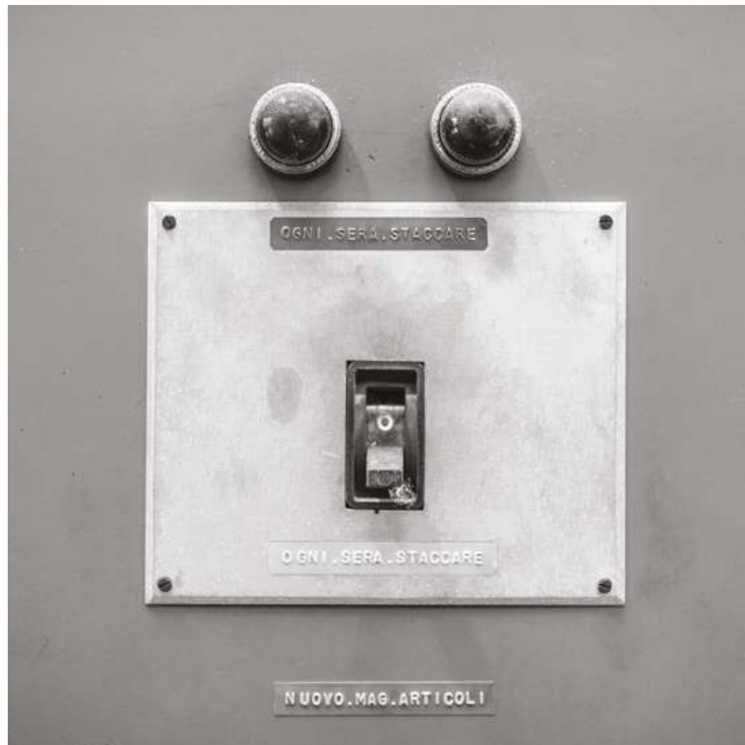
ANCHORED IN ITS INDUSTRIAL PAST
