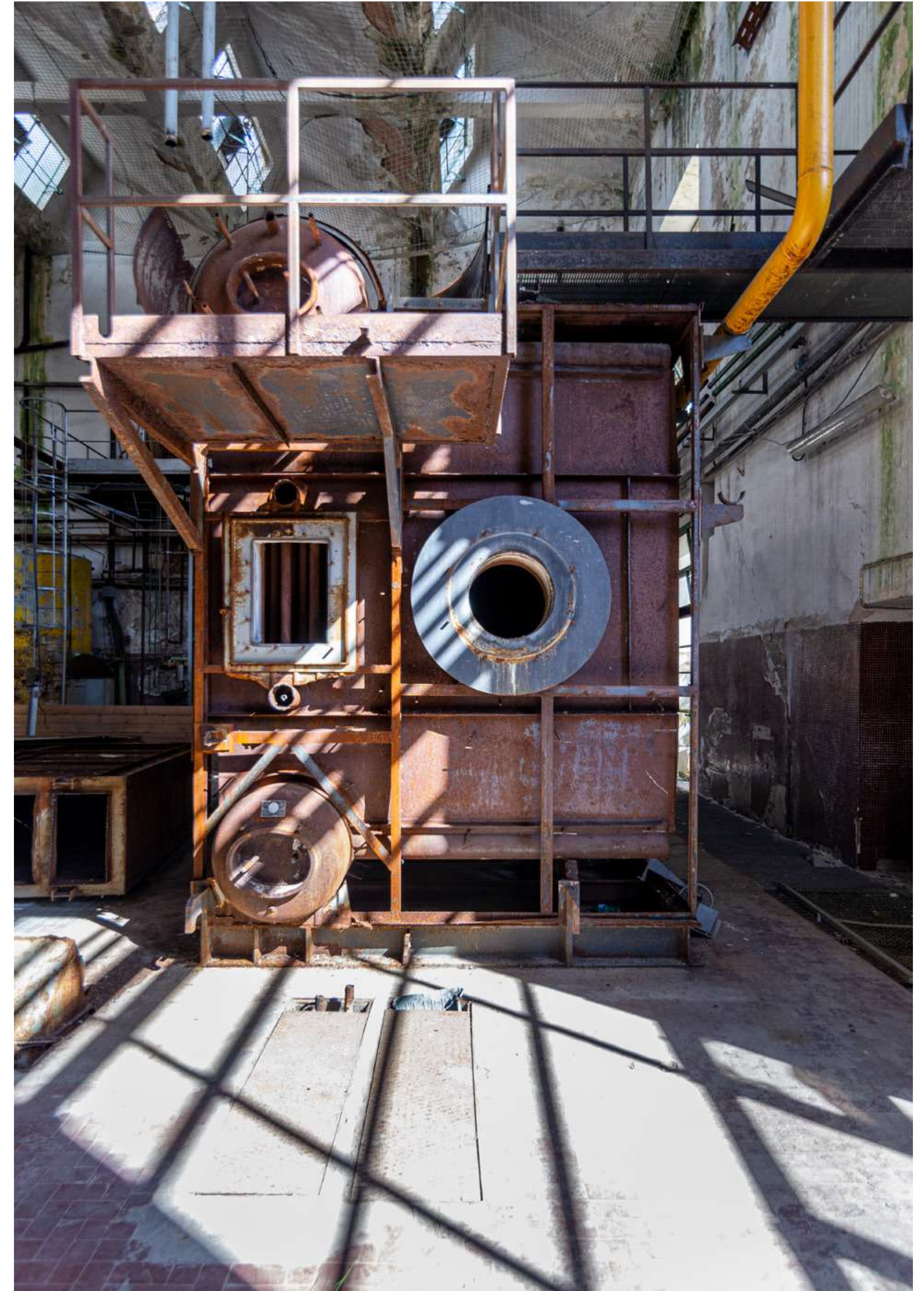
Industrial machinery, Building 10
