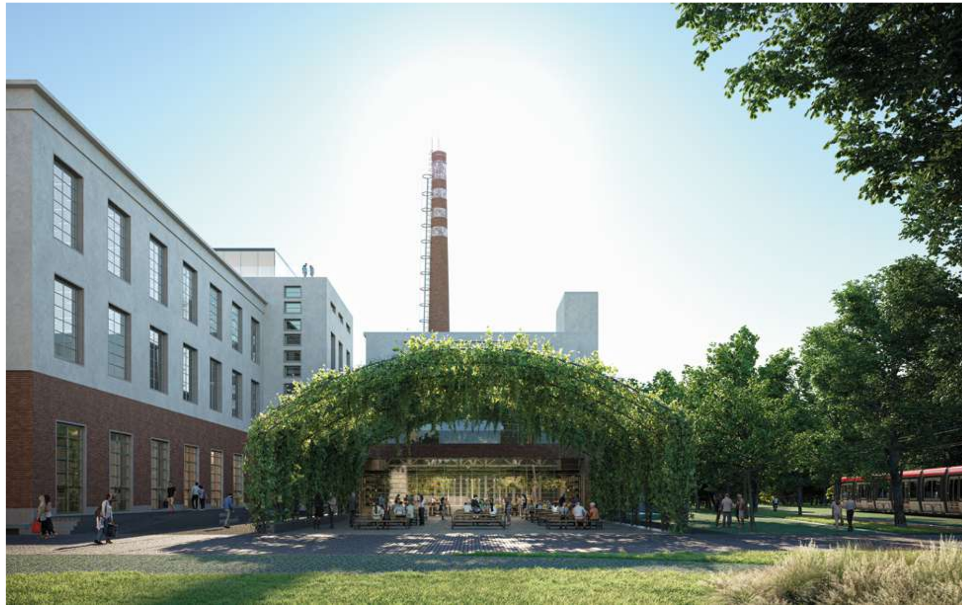
Building 10 External view
