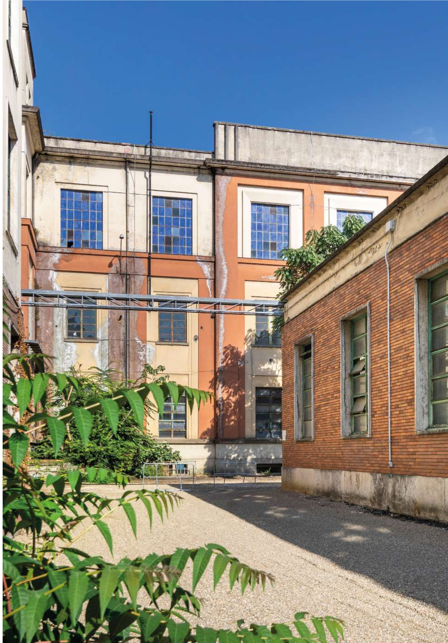
External View, Building 11
