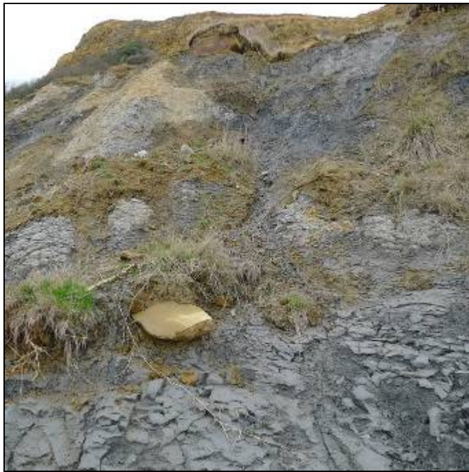
Plate 11. Unstable seepage line
