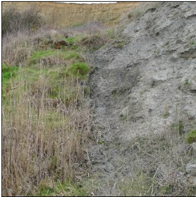
Plate 13. Small seepage line at Waypoint 669
