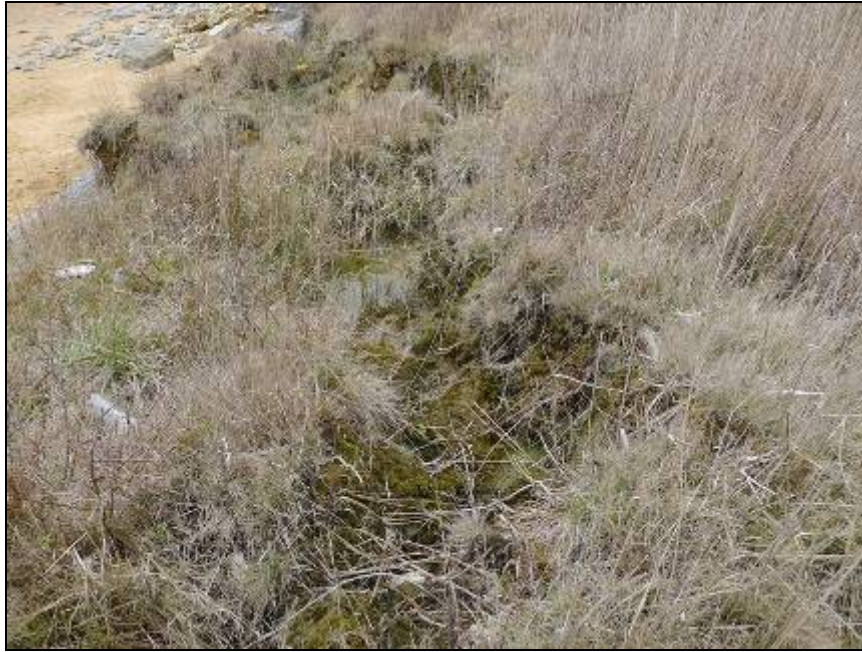
Plate 10. Perched marsh and rivulet near front of landslide
