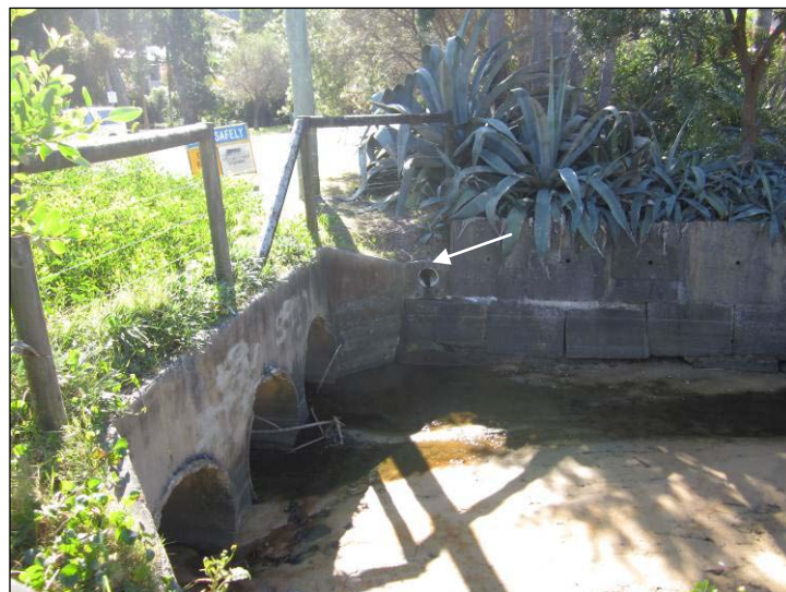
Figure 2-2 Culvert on lagoon entrance with arrow indicating entrance opening trigger
