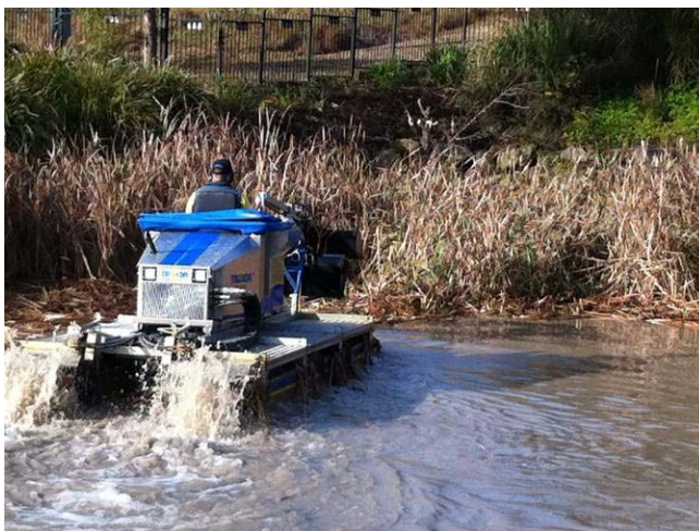
Figure 5-1 Amphibious machinery (e.g. TRUXOR) for sediment and weed removal/management
