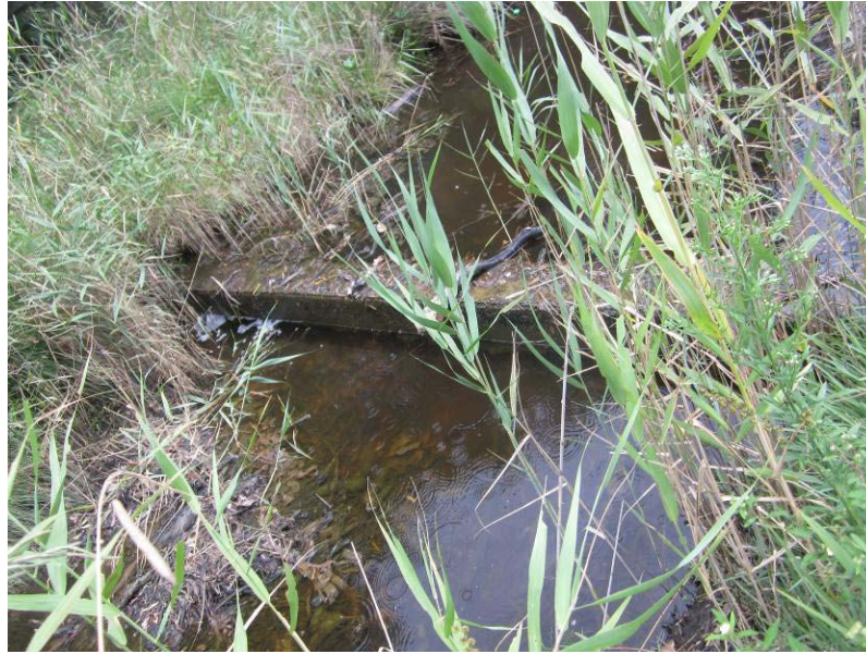
Figure 2-4 The weir on the entrance channel (photo taken March 2012)
